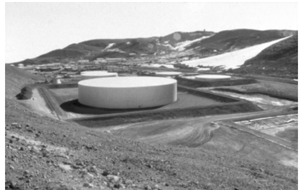
Storage tank for jet fuel at McMurdo Station
