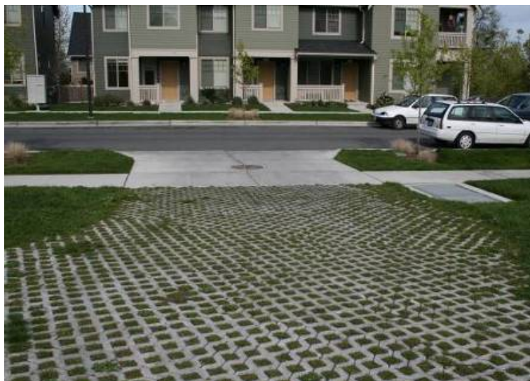
Figure 16 Example of permeable paving, Seattle. Photo: Maria Ignatieva
