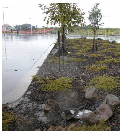
Figure 14 (Left) Swale, Auckland Netball Centre carpark with prostrate coprosma and treepits - boulders protect overflow grate that discharges to pond. Photo: Robyn Simcock.
