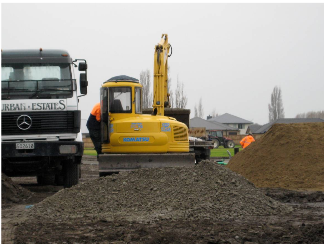
Constructing a New Zealand subdivision. Photo: Mark Hostetler
