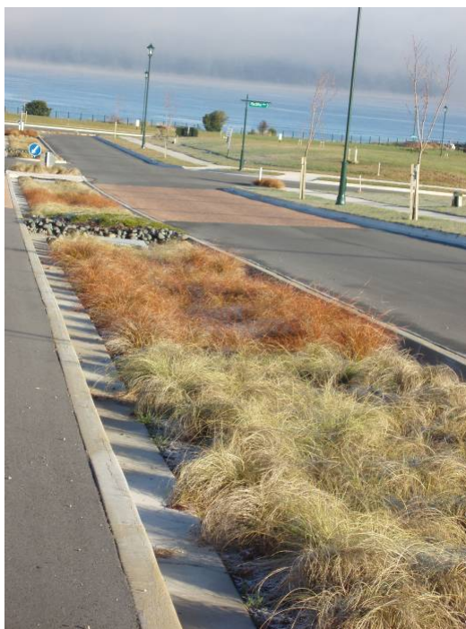
Figure 12 Carex cultivars cover swale surface at Wharewaka, Taupo. Note stone detention dams used to reduce flow strength. Photo: Robyn Simcock
