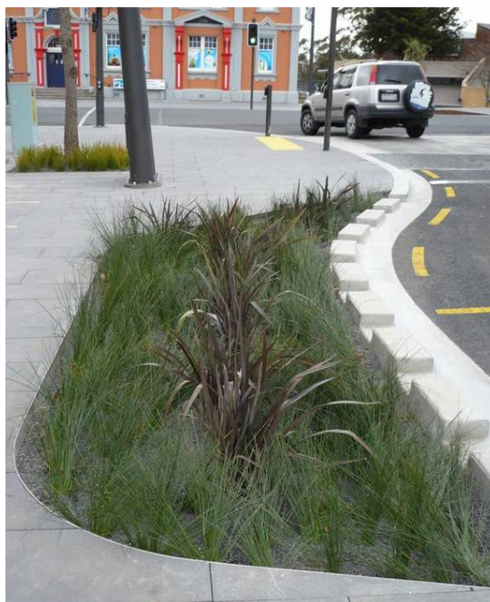
Figure 18 Hunt Street, Hamilton, raingarden associated with traffic calming (Megan Wraight, Wraight and Associates Landscape Architects). Photo: Robyn Simcock
