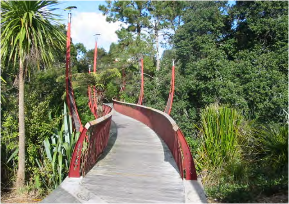
Figure 27: The Rewa Rewa footbridge across the Whau River connects the public with efforts to maintain the integrity of this ecosystem as sought through LIUDD principles and methods. Photo: M. van Roon
