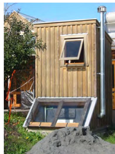
Figure 10: Clivus Multrum compost toilet at Earthsong, Waitakere City. Photo: M. van Roon
