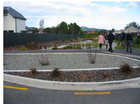
Figure 9: Addington, Christchurch. Alternative stormwater solutions - riparian restoration in background and raingarden in traffic island in foreground. Photo: M. van Roon
