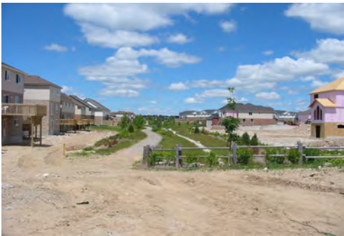
Figure 7: LIUDD mixed housing forms differ from traditional New Zealand single lots, offering greater expanses of shared open and amenity space and conserving natural areas by clustering homes and using vertical forms. Photo: M. van Roon
