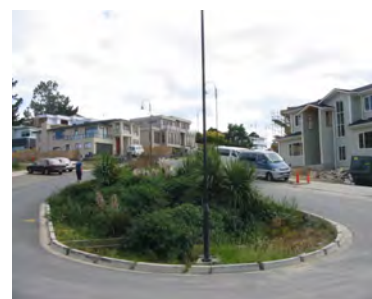
Figure 12: Biofiltration garden in centre of road. Photo: M. van Roon.
