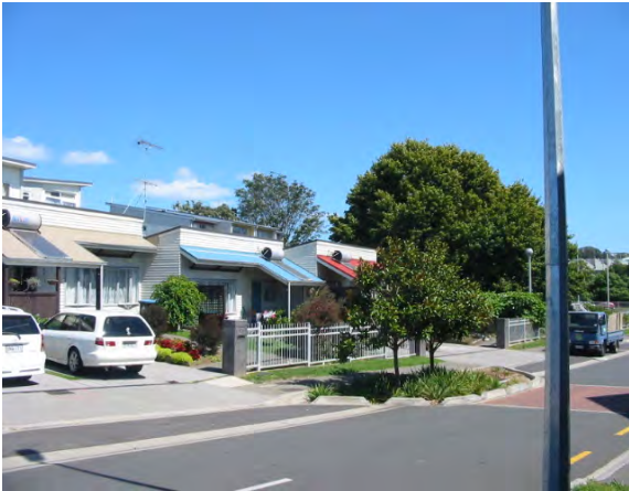
Figure 35: Small tenanted houses at Talbot Park with solar power, raintanks, and street-side raingardens. Photo: M. van Roon
