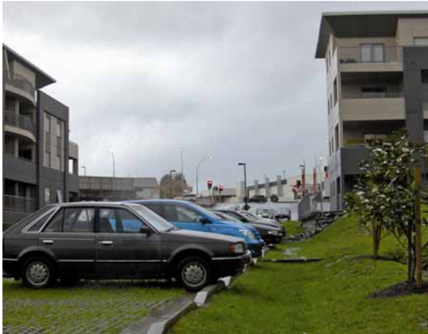
Figure 27: Permeable car park with discrete concrete blocks and mown grass between. Stormwater from the parking area runs into a grassed swale (centre). Photo: Robyn Simcock
