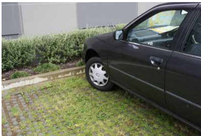
Figure 26: Concrete block permeable paving with mown grass, Morning Star Apartments, Auckland, New Zealand. Photo: Maria Ignatieva
