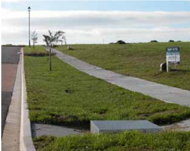
Figure 31: (Left) - Mown grass swale treating runoff from adjacent footpath (the grate covers the entry to a pipe taking water to an infiltration bed). Photo: Robyn Simcock
