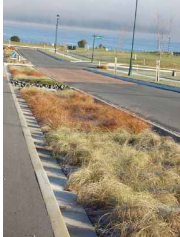
Figure 32: (Right) Carex cultivars cover swale surface at Wharewaka, Taupo. Stone detention dams reduce stormwater velocities and erosion during high runoff events. Note the absence of a curb; instead a drop discourages vehicle entry. Photo: Robyn Simcock
