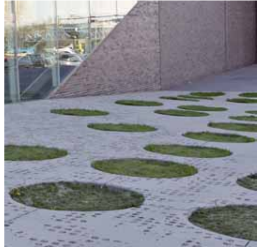
Figure 36: Mini-soakage areas (non-linear swales) with grass inset add interest to and reduce runoff from a large paved area outside an art gallery, Minneapolis, Minnesota, USA. Photo: Robyn Simcock
