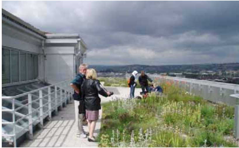
Glenn Stewart and Maria Ignatieva inspecting an extensive green roof in Sheffield, England where this will soon be a requirement for new commercial buildings. Photo: Colin Meurk
