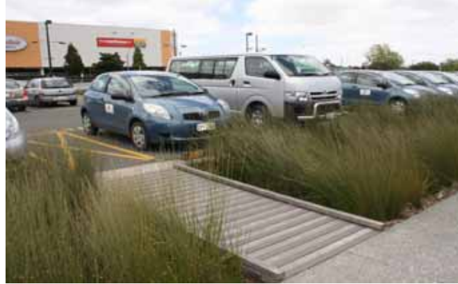
Figure 37: Bioretention strip planted mainly with oioi, rushes and other sedges. The wooden walkway covers an overflow structure. Waitakere City Centre car park, Auckland, New Zealand. Design: Meghan Wraight, Wraight & Associates. Photo: Maria Ignatieva
