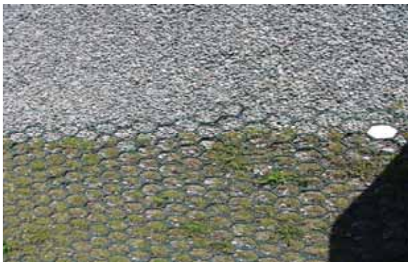
Figure 30 (a) and (b): Strong plastic grids increase bearing strength, reduce compaction of substrate, and allow plants to grow. Melbourne, Australia. Photos: Marjorie van Roon
