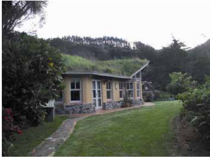
Figure 19: Extensive green roof on a private house in Matakana north of Auckland, New Zealand. Photo: Marjorie van Roon
