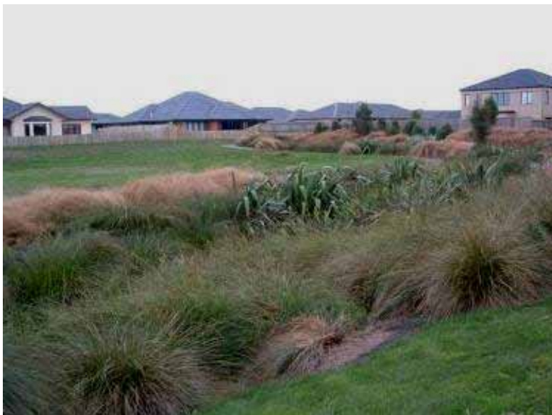
Figure 44: Vegetated swale and overflow detention and infiltration pond, Aidanfield, Christchurch. Photo: Colin Meurk
