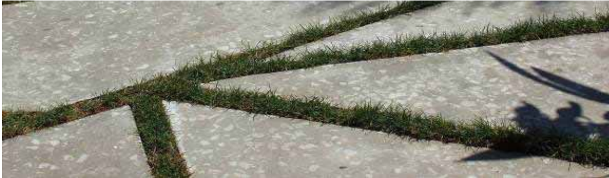
Figure 29: 'Friendly' concrete – relatively large gaps between pavers planted in grass or broadleaved groundcovers – reduces runoff. Photo: Robyn Simcock
