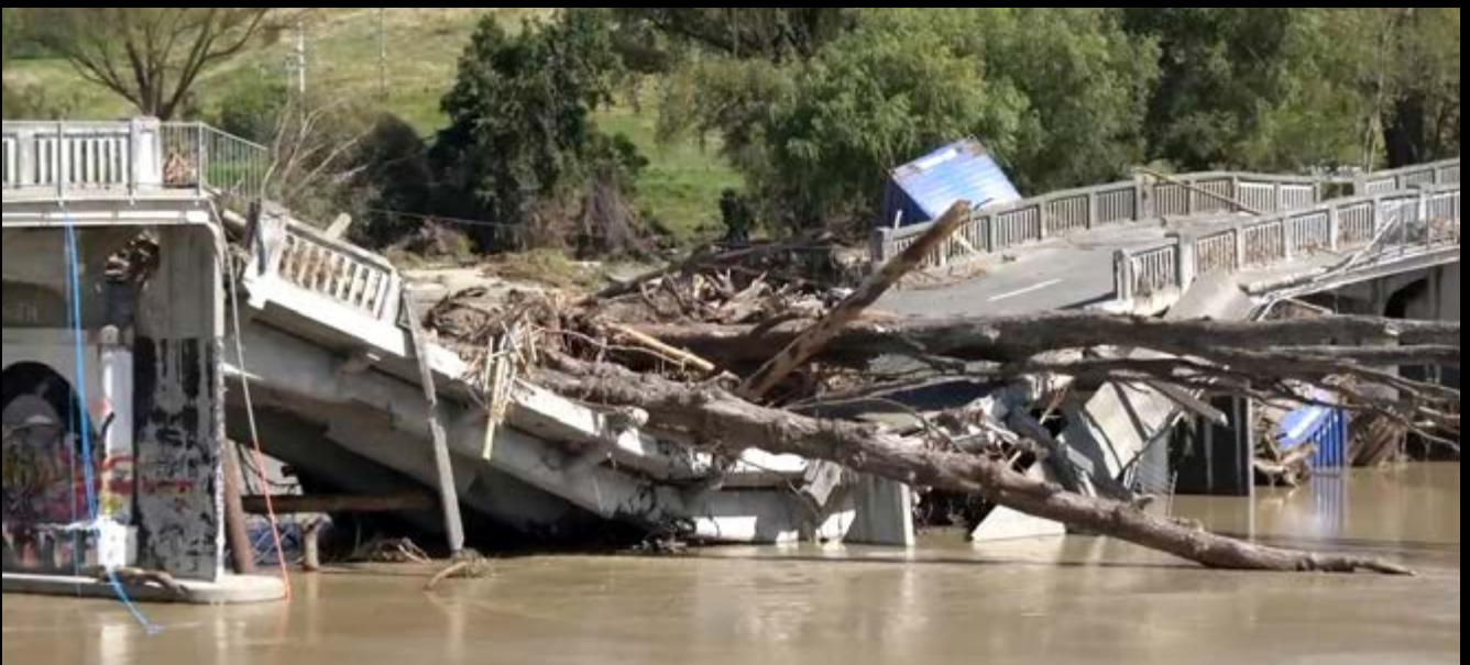
A bridge in the Hawkes Bay region damaged by slash brought down in Cyclone Gabrielle.
