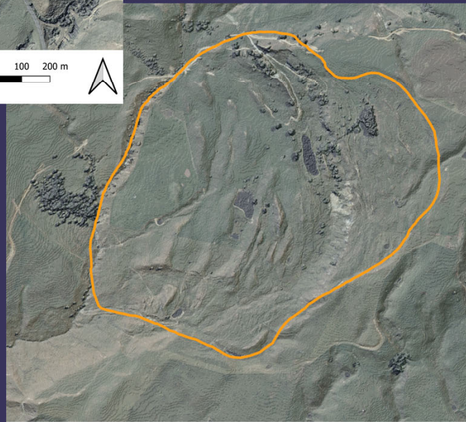
Example of an “Young” Landslide
