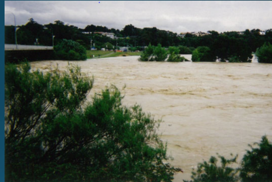
Manawatu Flood 2004 (Fitzherbert Bridge) –TAMIRO
