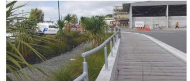
Native planting in retention basin, Pak 'n' Save, Wainoni Road
