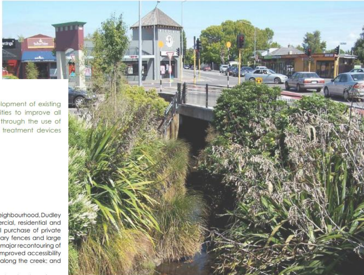
Plant to carpark in suburban centre, Hills Road, Dudley Creek
