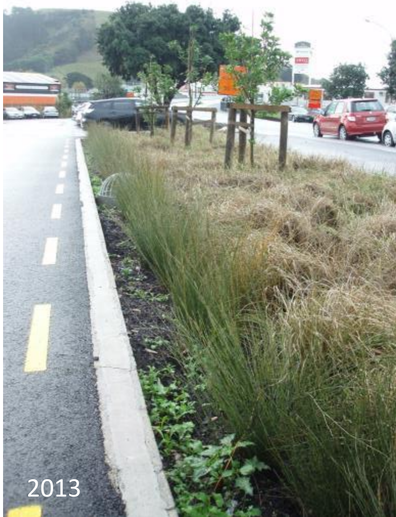
Site 5. Seamless integration of pre-existing trees within rain garden (left); location of overflow near edge allows efficient checks; bare areas should be replanted and re-mulched to avoid ongoing spraying. Right photos show expensive rain gardens – one carpark wide creates a long area of edge to maintain relative to treatment area and greater damage to trees: one larger rain garden would be more cost effective
