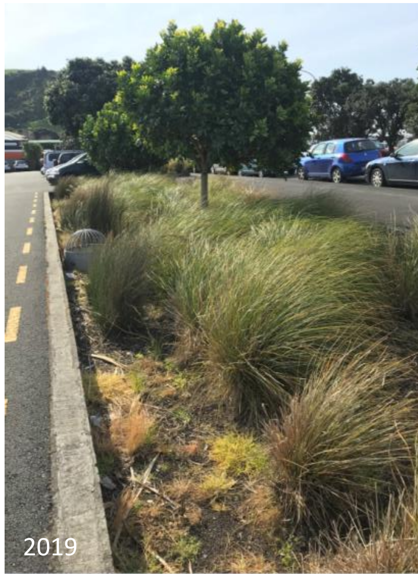
Site 5. Seamless integration of pre-existing trees within rain garden (left); location of overflow near edge allows efficient checks; bare areas should be replanted and re-mulched to avoid ongoing spraying. Right photos show expensive rain gardens – one carpark wide creates a long area of edge to maintain relative to treatment area and greater damage to trees: one larger rain garden would be more cost effective
