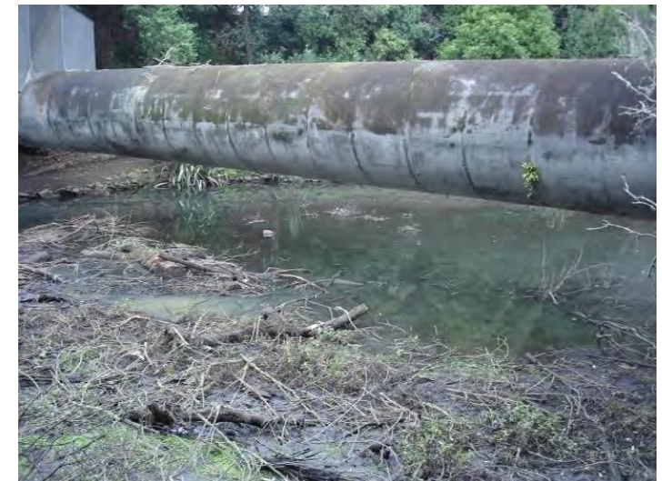
Eastern interceptor prior to AMETI
