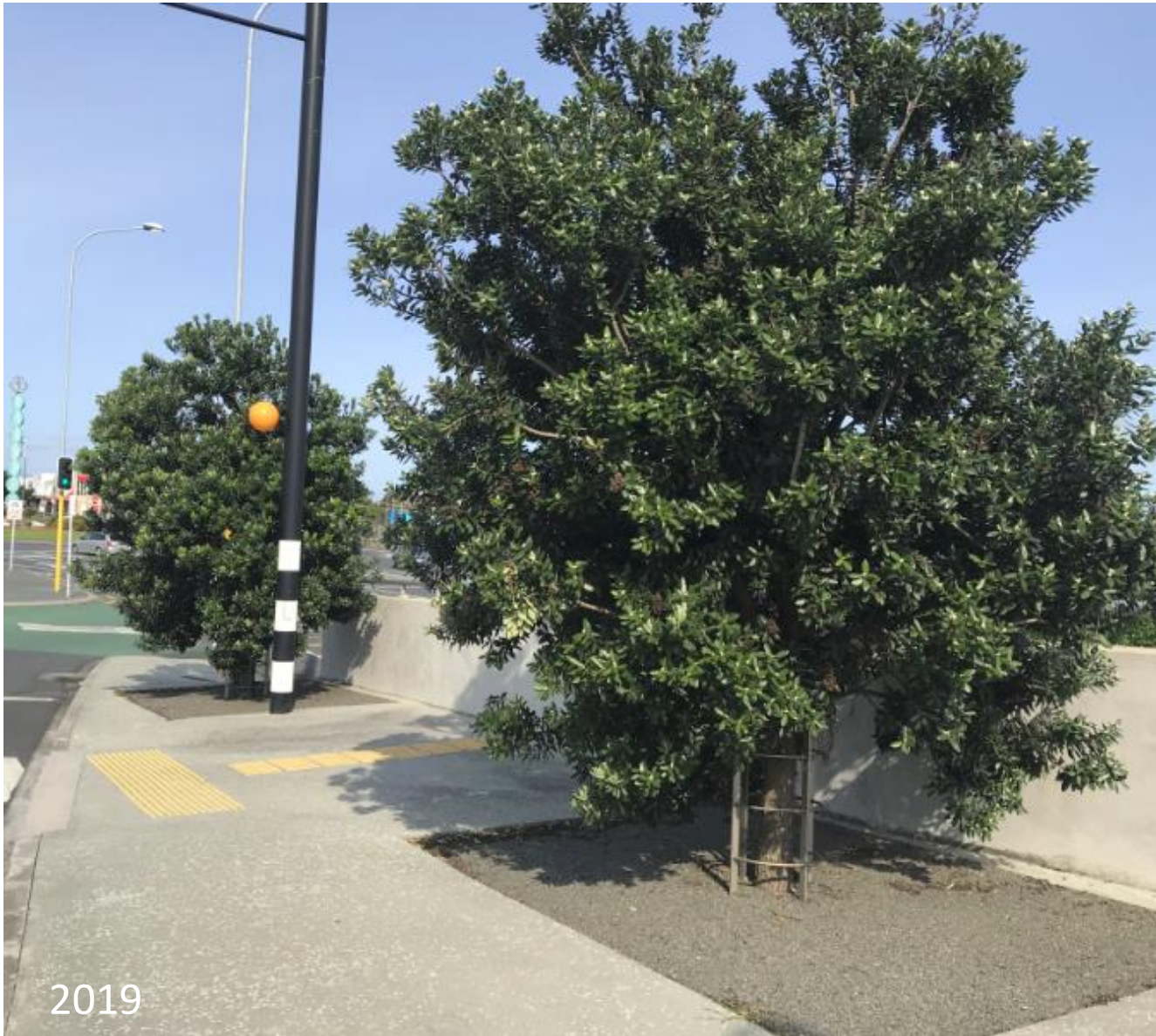
Site 6. Tree pits in overbridge with permeable paving (poured-in-place resin-bound pebbles). Resin must be kept away from the trunk or it 'ring-barks' the tree; use inner ring and loose gravel.
