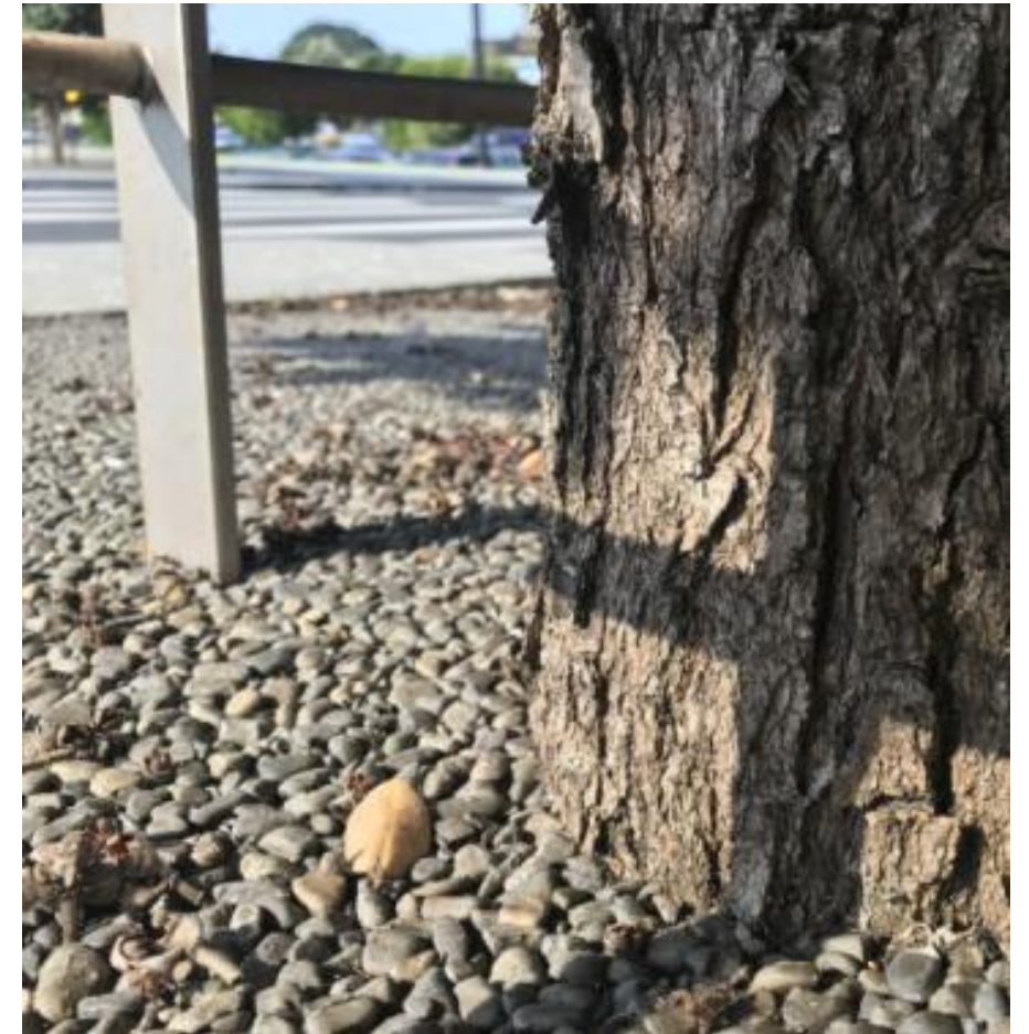
Site 6. Tree pits in overbridge with permeable paving (poured-in-place resin-bound pebbles). Resin must be kept away from the trunk or it 'ring-barks' the tree; use inner ring and loose gravel.
