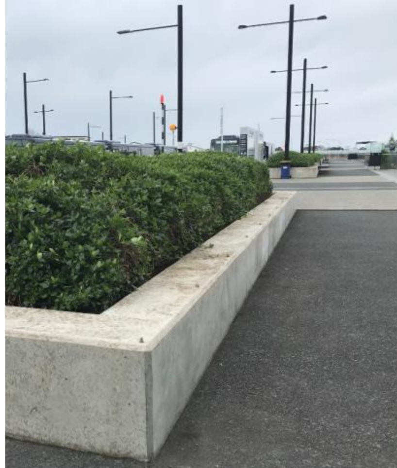
Site 2. Raised roadside planters on Quinlan Street do not receive stormwater so require irrigation (and its maintenance). Trimming at ground level (right) reduces weed invasion and litter input but prevents seating.
