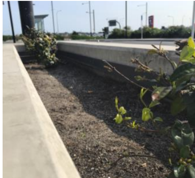
Site 2. Plants in narrow, raised planter boxes have died and need replacing with new mulching
