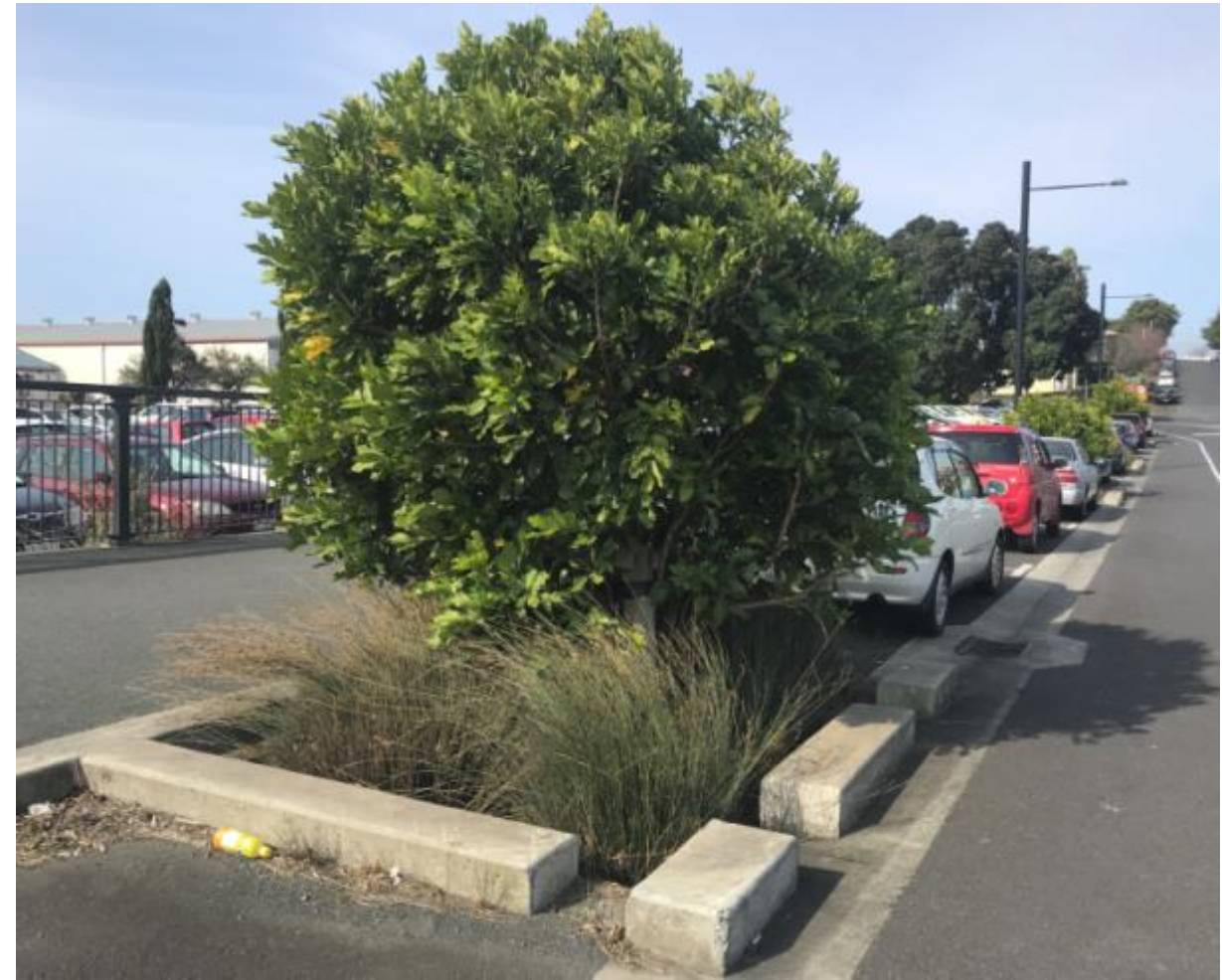
Site 4. Potaka Lane roadside tree pits with oioi groundcover and kohekohe trees shortly after establishment in 2013 and in late 2018
