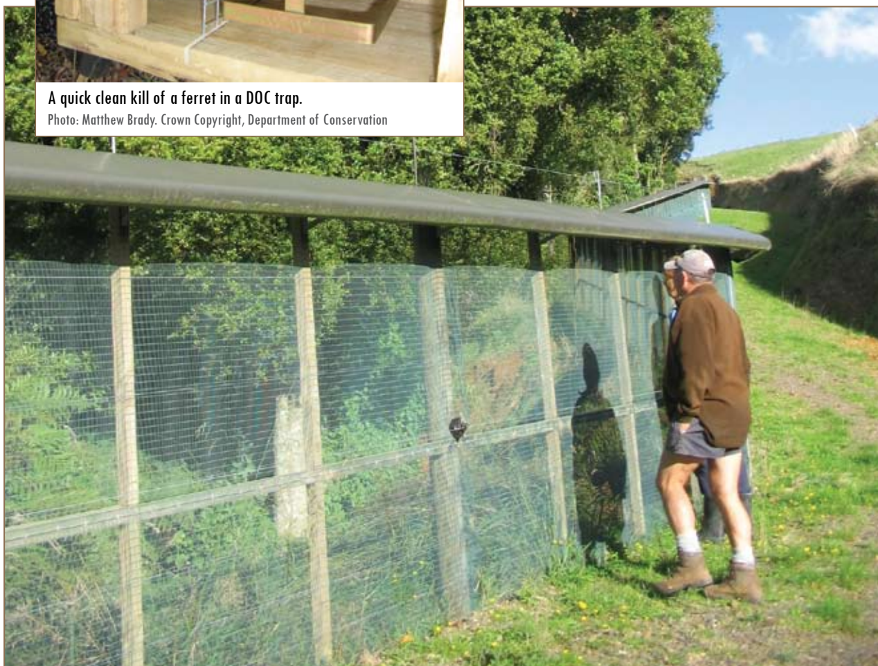
A section of the 42-km pest-proof fence at the Maungatautari Ecological Island, Waikato. Photo: Monica Peters, NZ Landcare Trust
