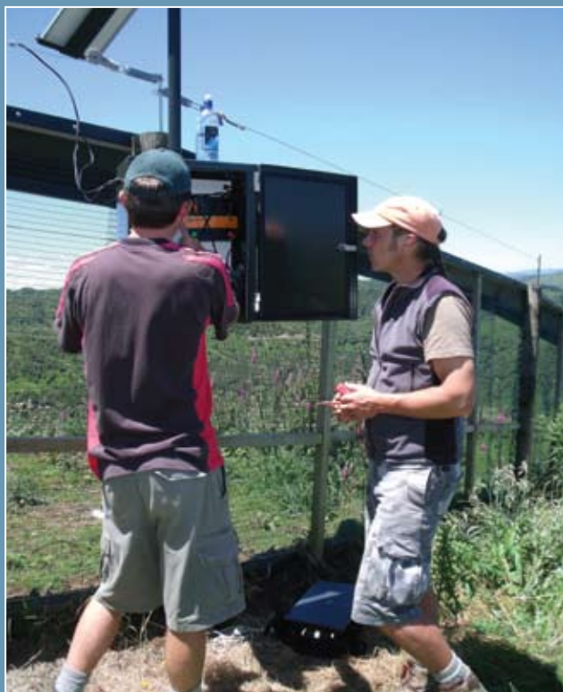
Fixing fence surveillance equipment. Photo: Rotokare Scenic Reserve Trust
