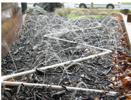
Layout of pipe aims to irrigate most of the available surface area; in 12 months it will be hidden by plants.
