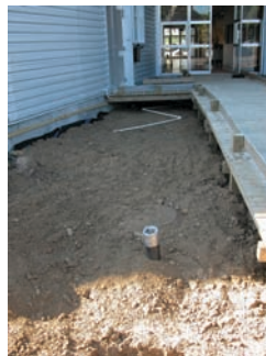
The flume that measures flow from the base of the raingarden. Topsoil spread.
