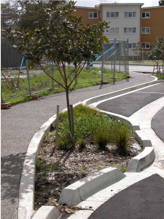
Rain gardens were designed to help slow traffic and provide visual amenity to Talbot Park, as well as detain and treat road runoff. Evergreen magnolias and native groundcovers of sedge, mountain flax and NZ iris were planted. Photo: May 2006, soon after construction.
