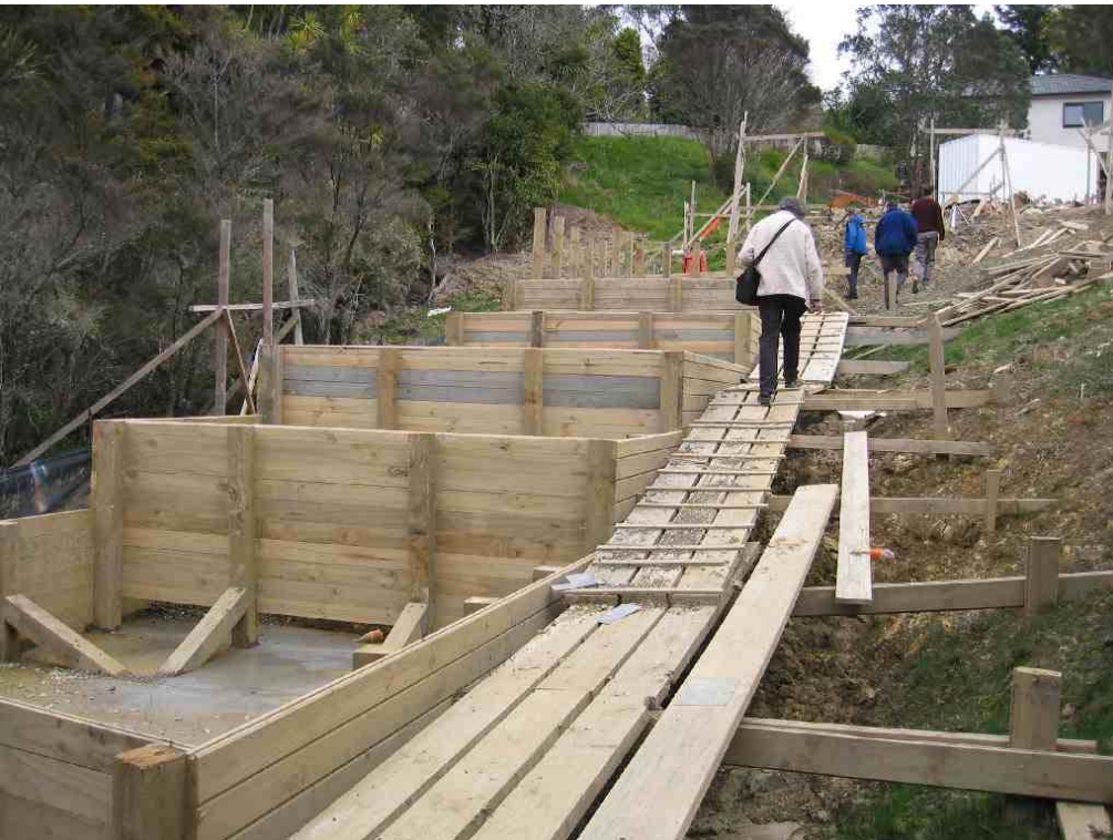
Photograph 5: Runoff treatment structure (under construction) at Verbena Road
