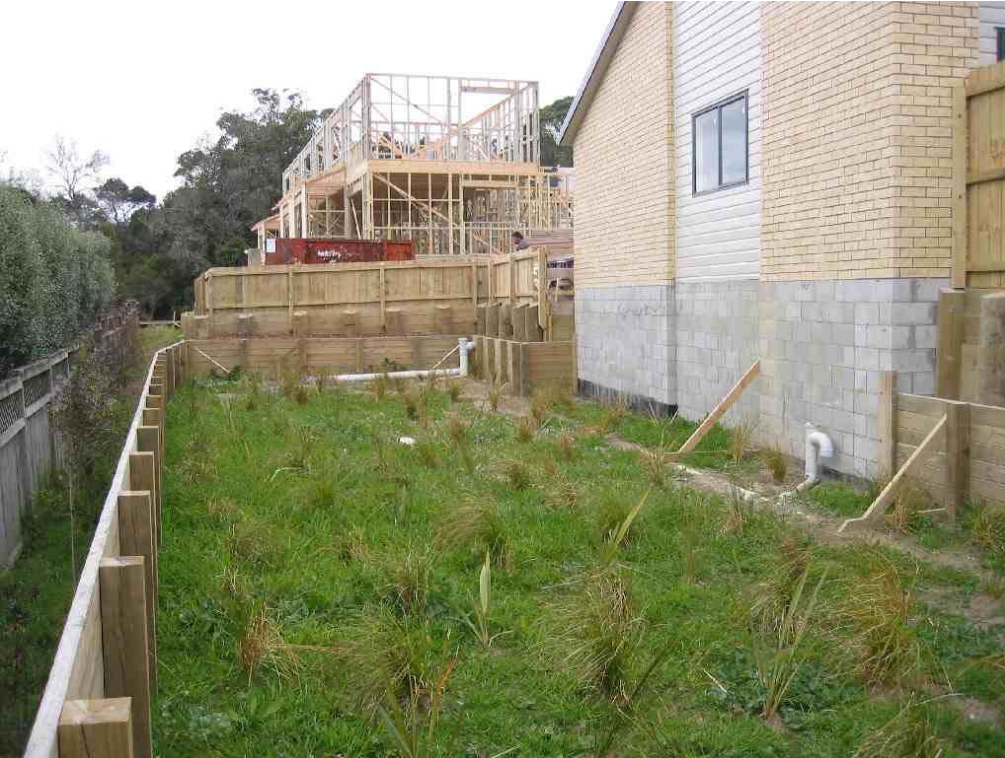
Photograph 4: Raingarden (under construction) for treating road runoff at Verbena Road
