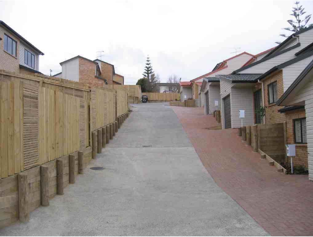
Photograph 6: Highly impervious surfaces around houses have resulted at Verbena Road
