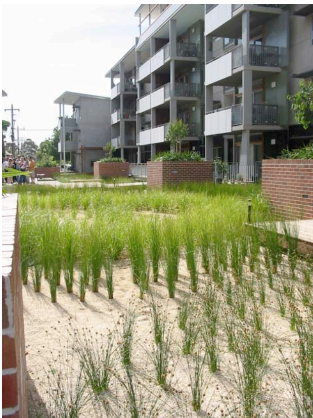
Photograph 8 Cremorne Street, Melbourne. Retrofitted biofiltration beds in brownfield street.
