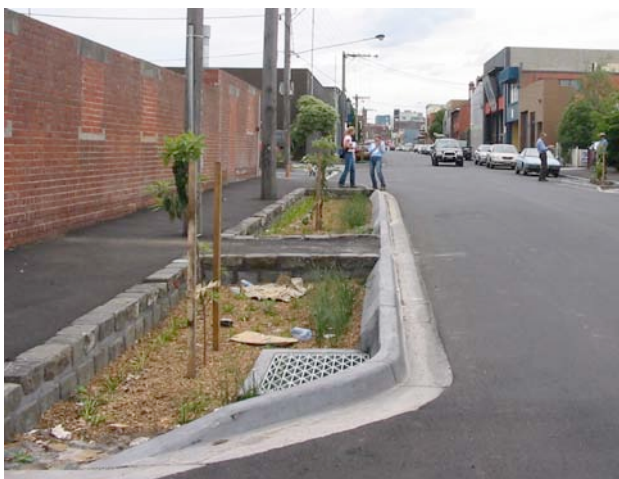
Photograph 8 Cremorne Street, Melbourne. Retrofitted biofiltration beds in brownfield street.
