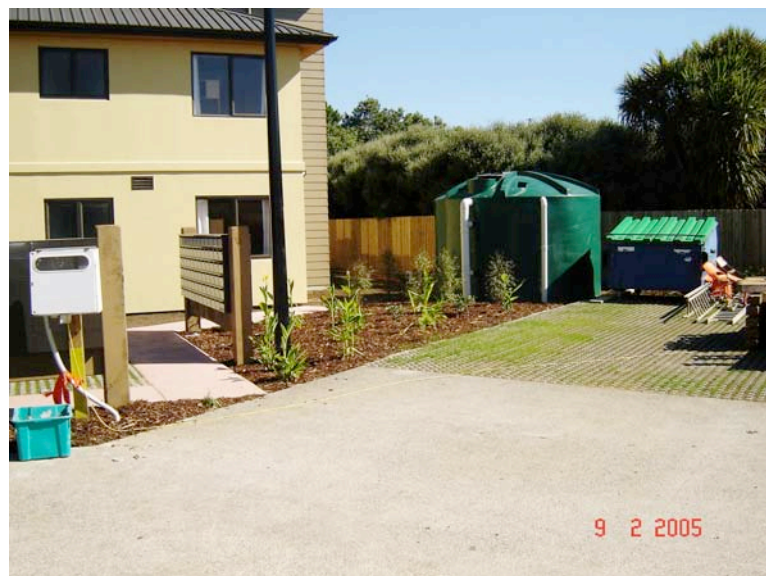
Photo 2 Example of Permeable Areas and a Rain Tank, Glenfield (photo courtesy of Peter Nagels)
