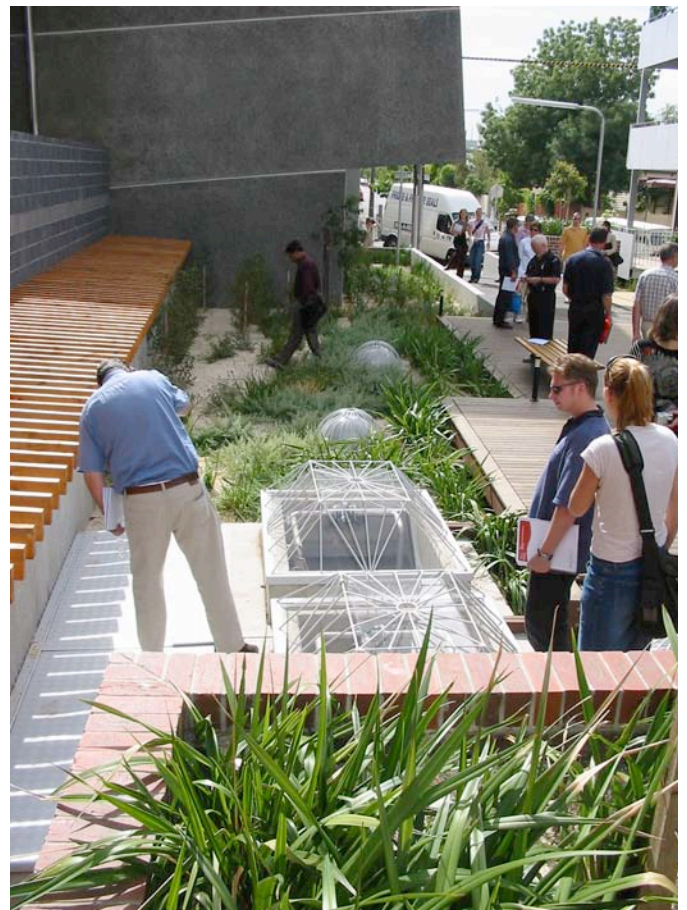
Photo 5 Transparent Greywater System Observation Dome on Inkerman Site
