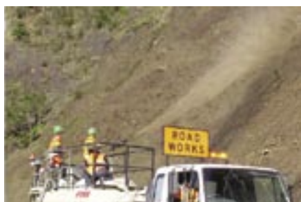
Hydroseeding moss mixture onto a slip face in the Manawatu Gorge.
