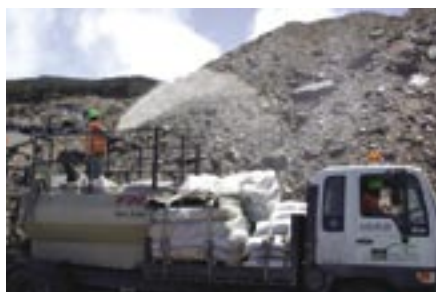
Hydroseeding moss mixture onto a bouldery sandstone waste-rock-dump slope at Stockton Mine.
