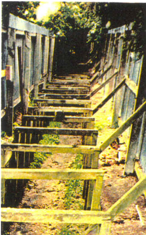
A fenced off timber-lined drain – no natural margins for this stream (CCC NPGU)
