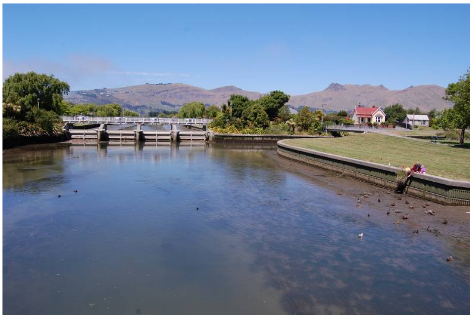
The Woolston Barrage
