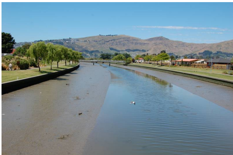
The Woolston Cut looking downstream from the barrage, 2008
