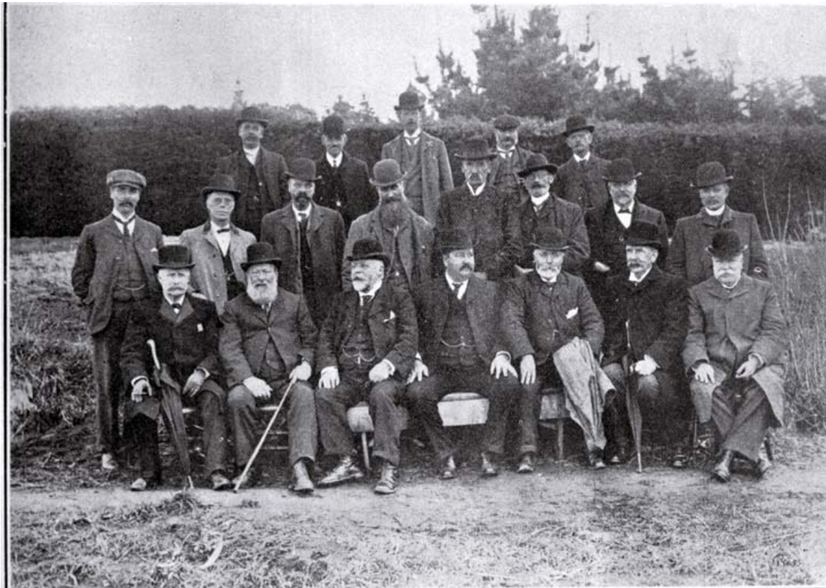
Members of the Christchurch Drainage Board and visitors present at the opening of the septic tank, Bromley, 4 September 1905 (CCC NPGU)
