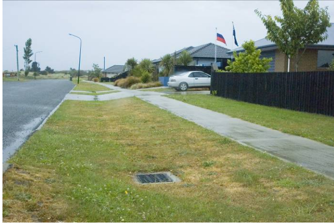
Roadside swales with subsoil drains: a system that collects and cleans stormwater and controls groundwater levels
