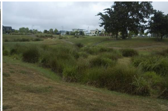
Wetland stormwater treatment and basin, Redwood
