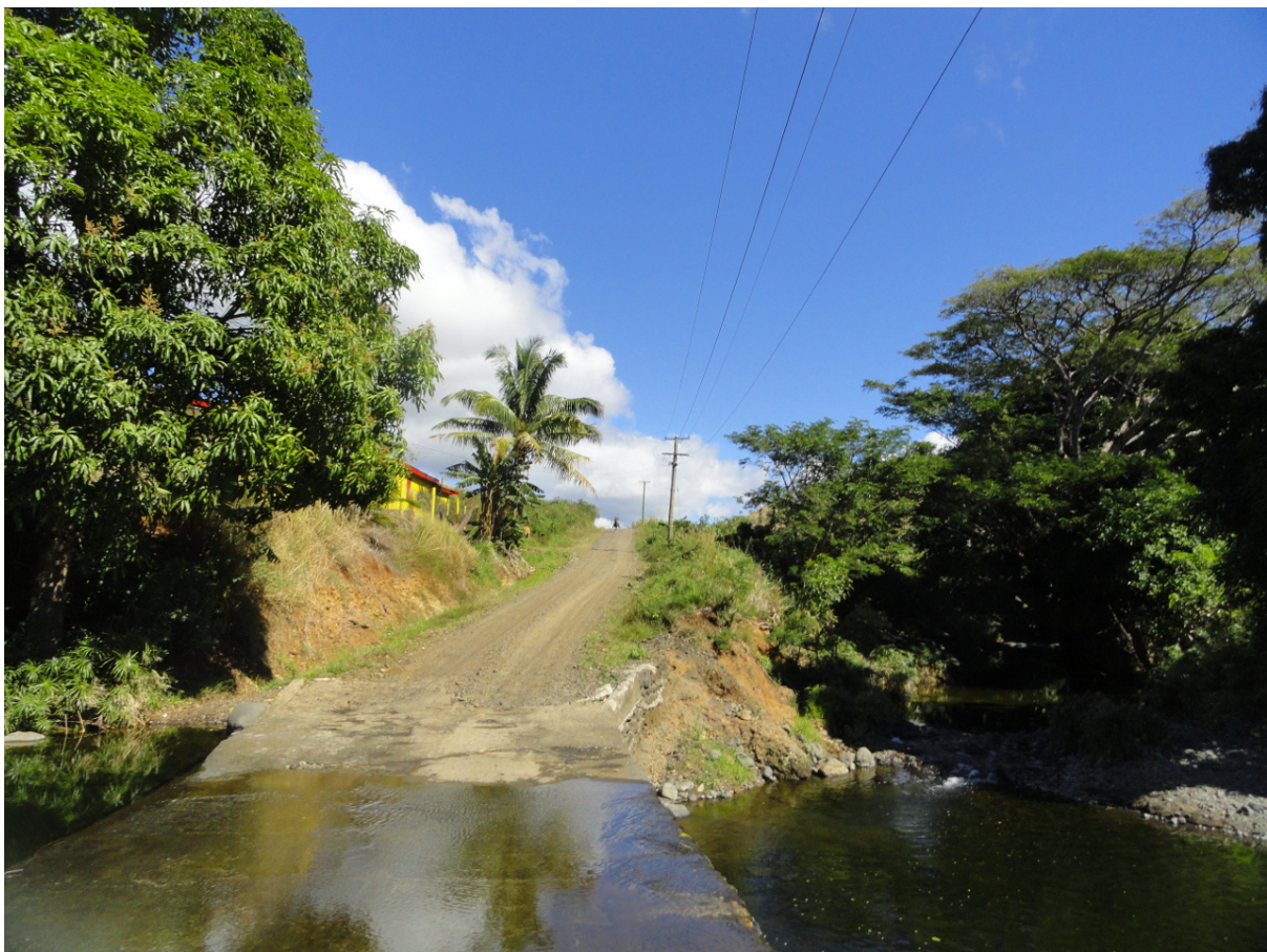
Crossing on a tributary of the Ba River.
