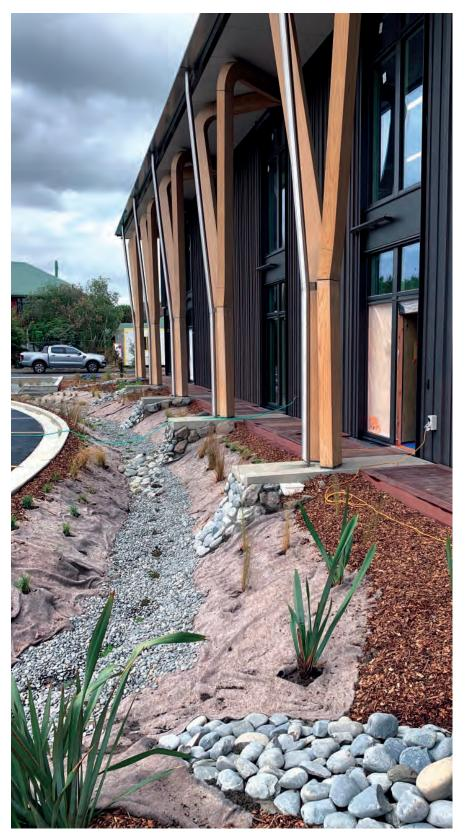
Rainwater from the office wing of our Te Rauhītanga building is channelled into a rain garden. We will harvest water from the main office roof for use in the building.
