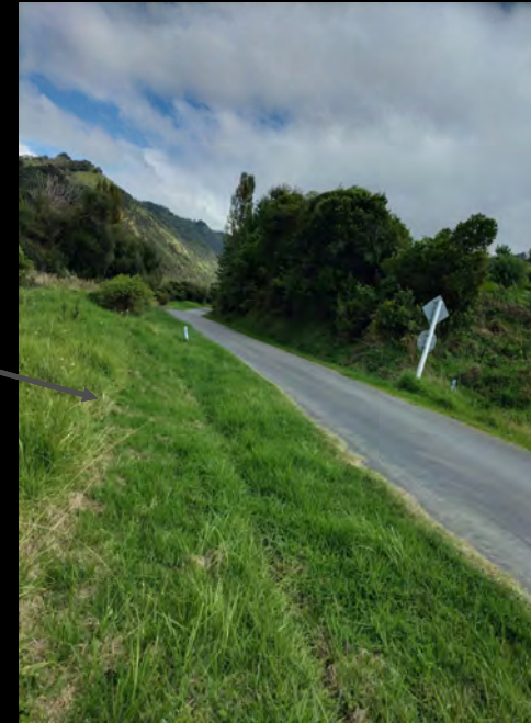
Ngāti Hau, Hiruharama ūrupa, instability, erosion at side of river
