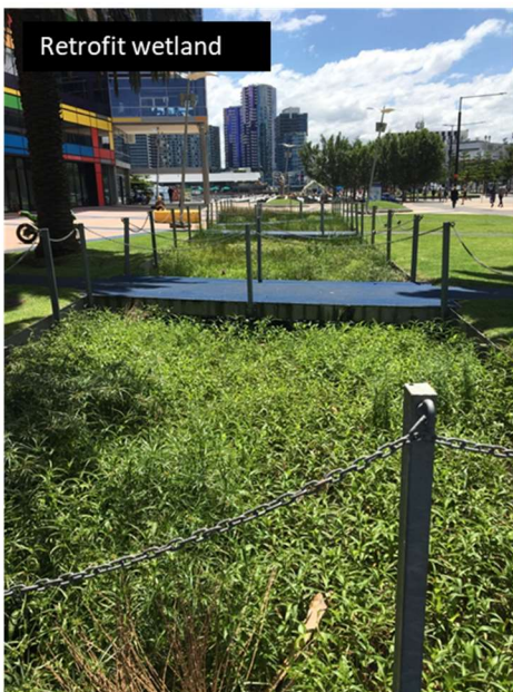
Retarding basin and biofiltration system
