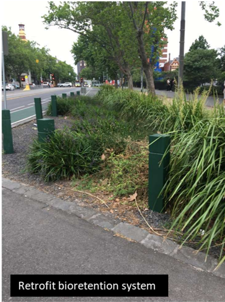
Tree pits and biofiltration systems
