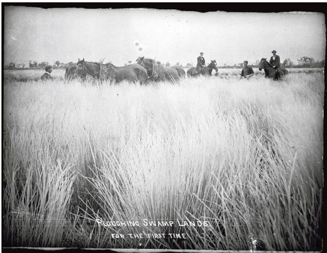
FIGURE 1 Ploughing swamplands for the first time c1890s (Photo: Palmerston North City Library Archive)
