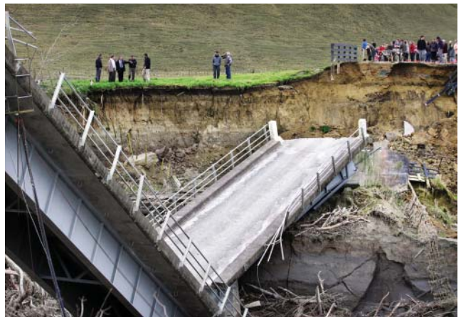
Downstream effects of flooding – Ngaturi Bridge on the Mangawhero River, July 2006 (photo courtesy of Manawatu Standard)
