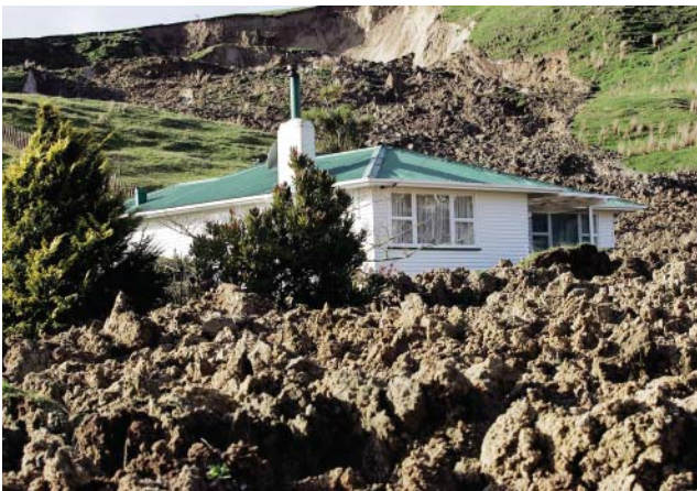
Catastrophic effects of hill country erosion in the Rangitikei River catchment, July 2006 (photo courtesy of Manawatu Standard)
