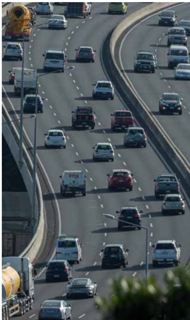
Newmarket overpass, Southern Motorway, Auckland
